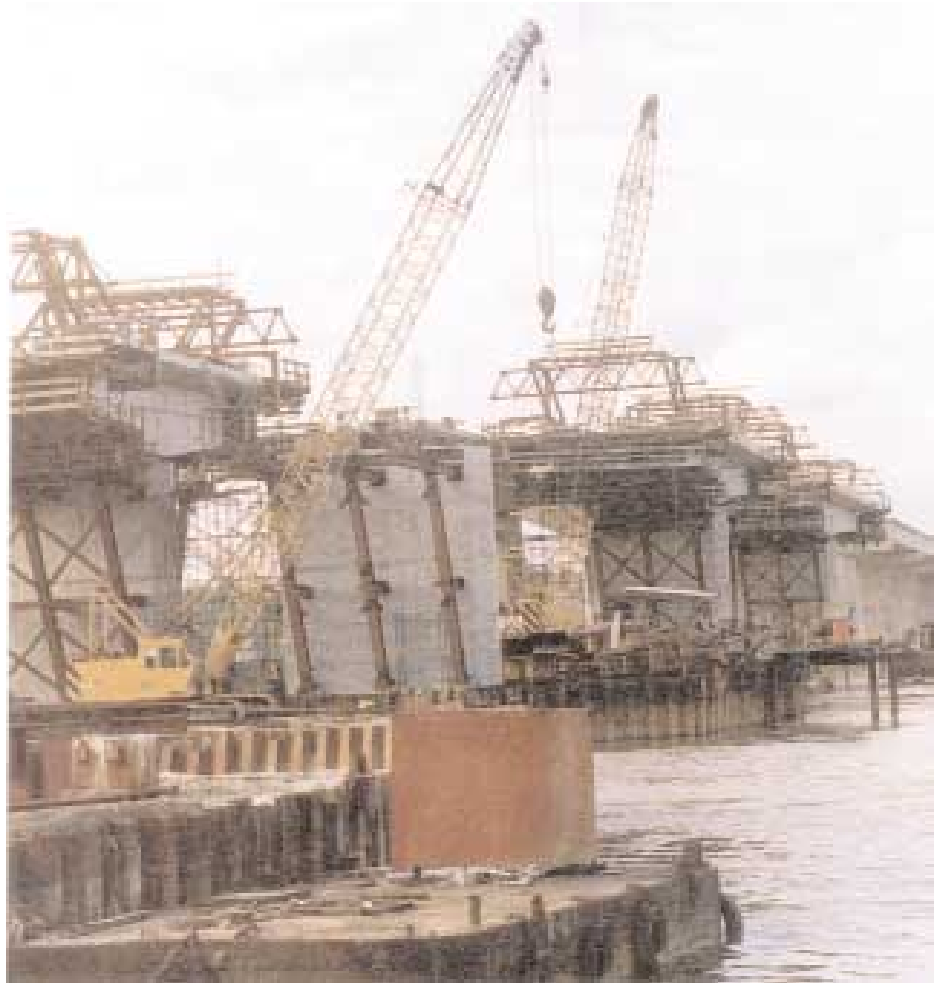
Cantilever segmental construction of the main spans.
