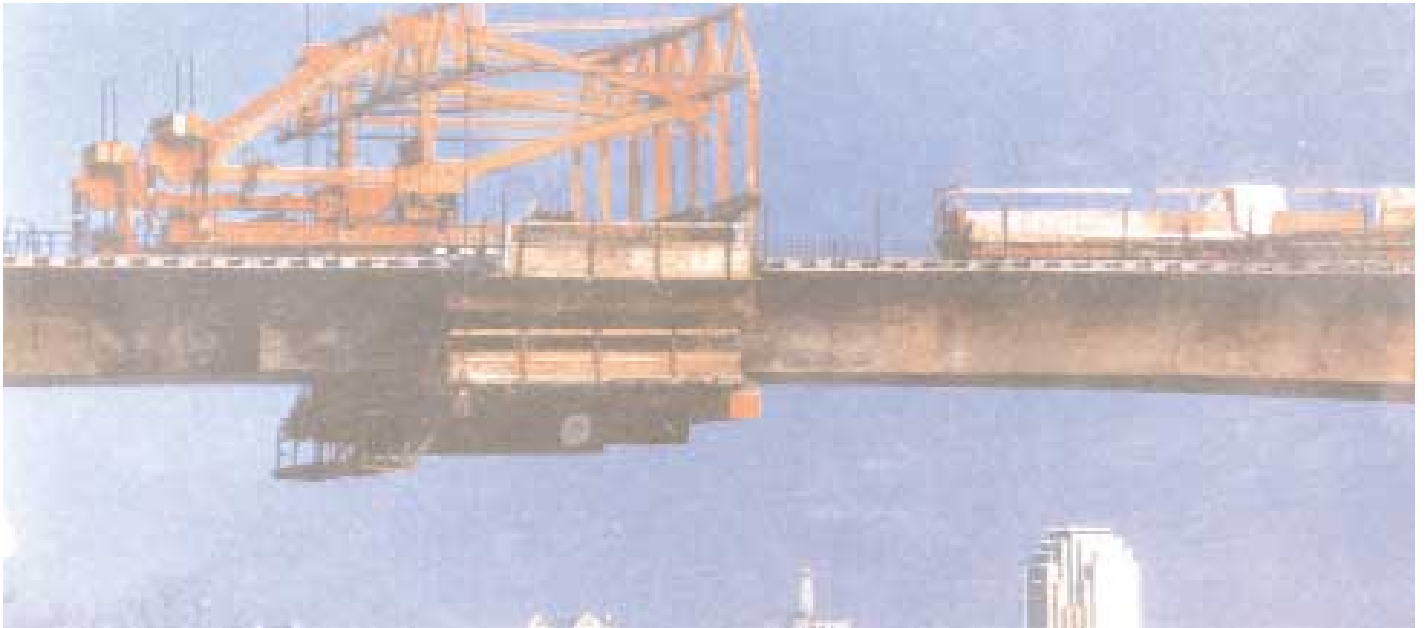
Westmoreland Bridge under construction in Dallas, Texas.
