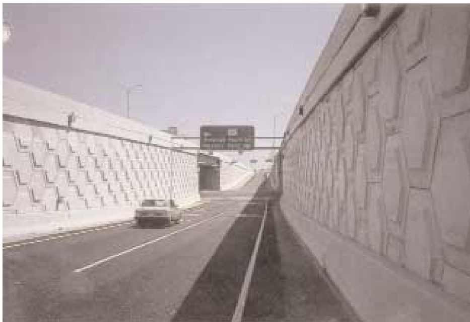
Retained Earth walls provide visually interesting access ramps to 1 - 275 south of Tampa, Florida.
