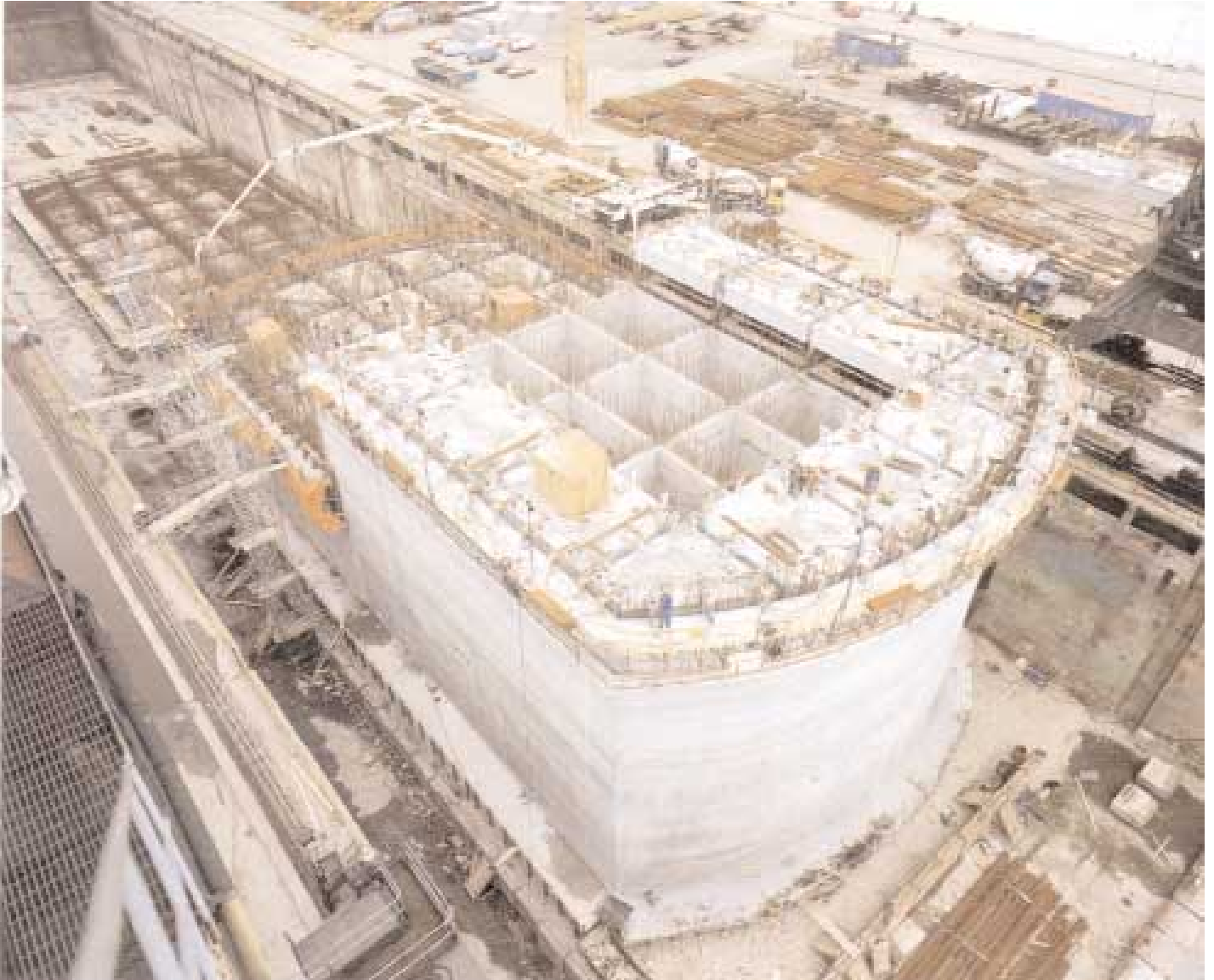
Slipforming of the first Dartford Bridge caisson.
