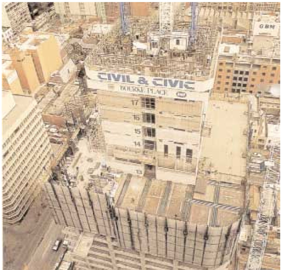
Bourke Place climbform at level 18 with post-tensioned floors at level 13.
