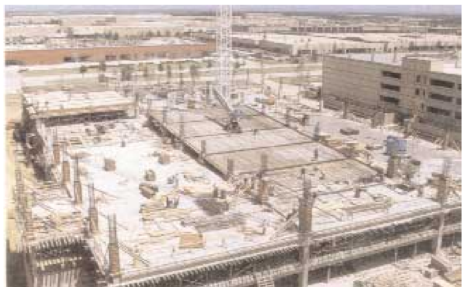
American Airlines parking expansion utilizes more than 460 tons of prestressing strand.
