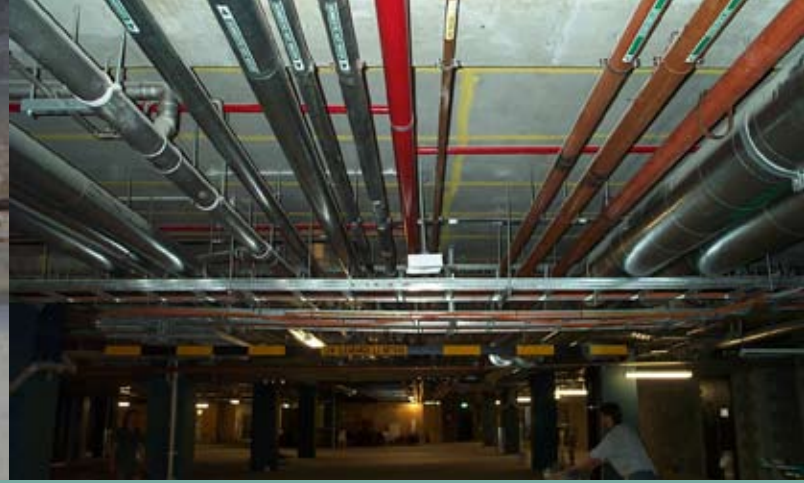
▲ Slab markings identify tendon locations
