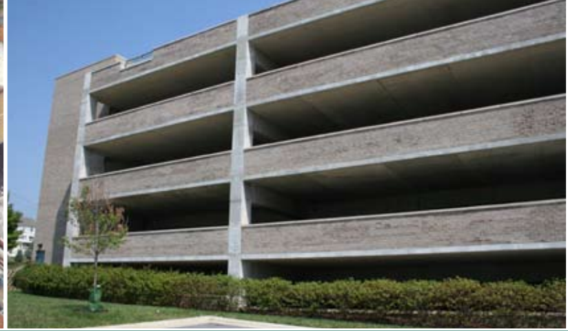
▲ Post-tensioned parking structure
