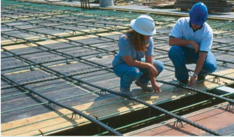
▲ VSLAB+® Bonded Slab tendons in flat plastic ducts
