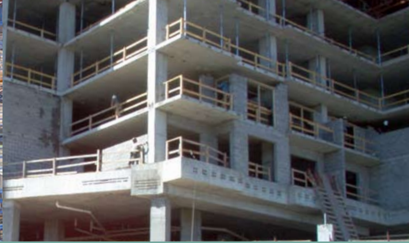
▲ Post-tensioned slabs, transfer plates and beams
