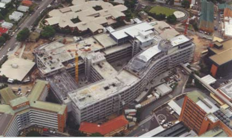
▲ Post-tensioning provides design flexibility
