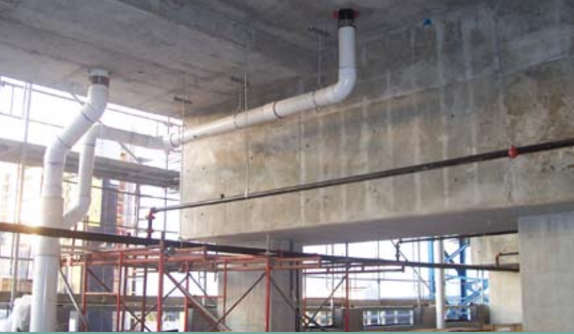
▲ Large transfer beam with bonded multistrand post-tensioning
