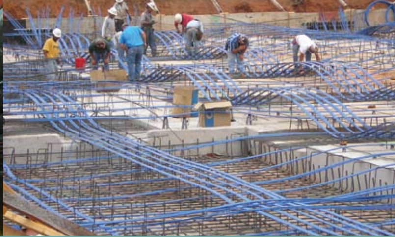
▲ Post-tensioned mat foundation construction
