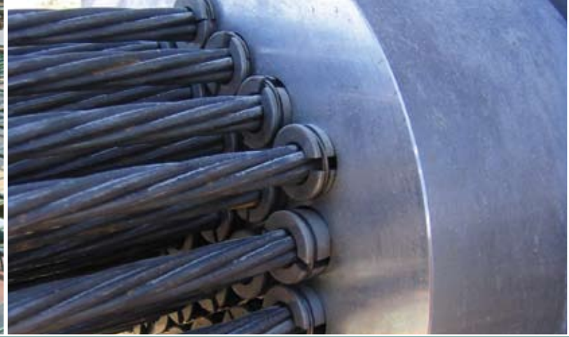
▲ Bonded multi-strand post-tensioning system
