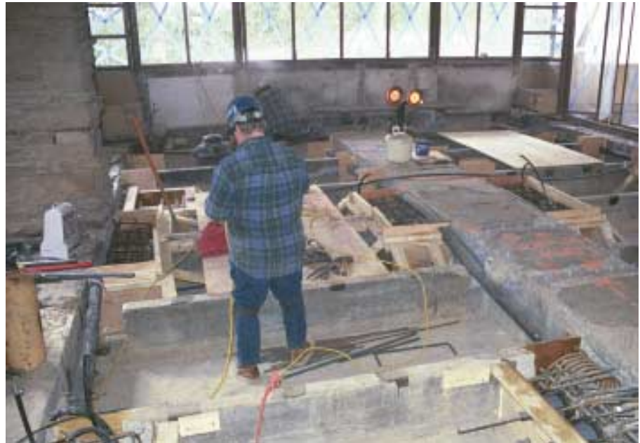
Fig. 2: One of the primary girders at the main level that cantilevers over the stream and supports the south parapet wall (background). Note the four structural window mullions at the parapet and the dead-end anchorages with spiral reinforcement and grout vents (foreground)
