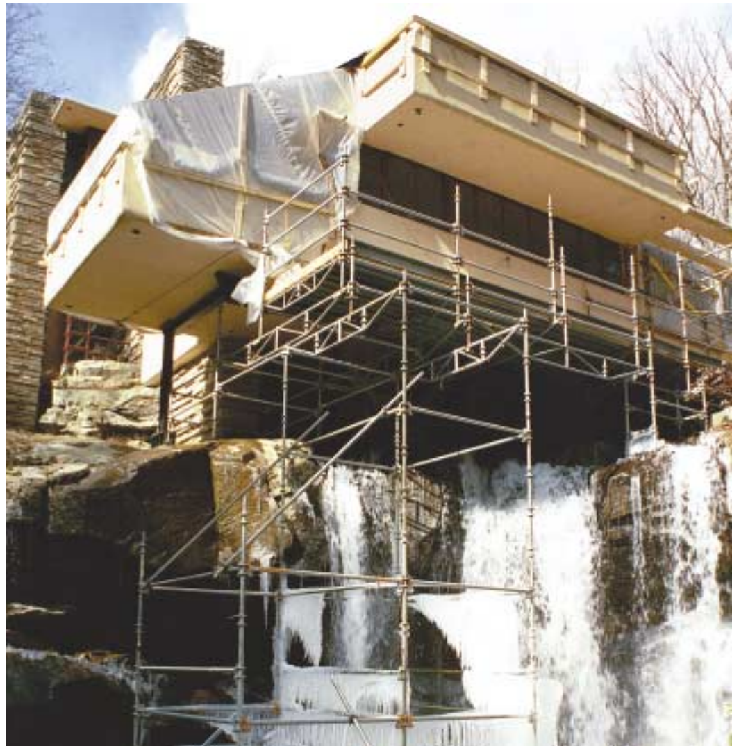
Fig. 1: View looking up at Fallingwater from stream below. The home is comprised of a series of concrete cantilevered trays. From downstream, water appears to pour out of the structure
