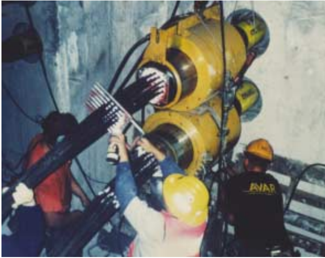
Tendon jacking for the SR 520 Evergreen Point Floating Bridge Rehabilitation
