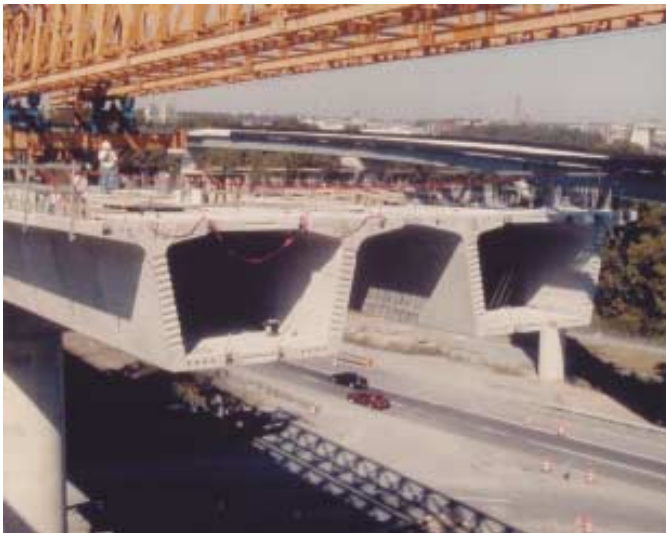
Segment erection on the Route 895 Connector/Pocahontas Parkway
