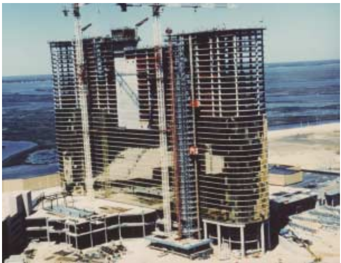
Borgata Hotel Casino and Spa under construction
