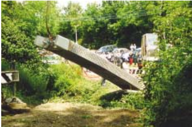
Fig. 3: Tring Bridges, Tring, UK
